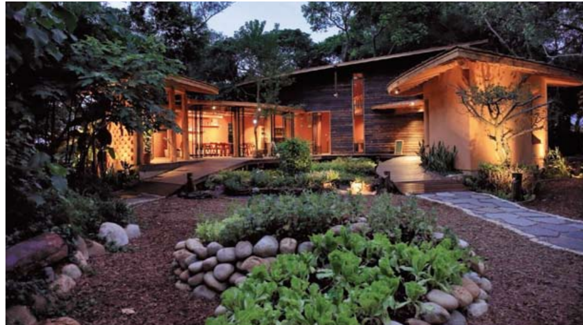
"An Eco-friendly Home for Four" at the Houli Ranch and Forest Site is the first sustainable building in Taiwan to use rice straw as wall filling material.
