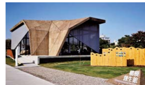
Fengyuan Huludun Park Expo Site’s Entrepreneurship Pavilion
