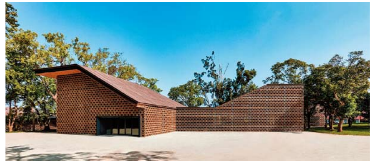
Discovery Pavilion is the main exhibition hall of Houli Horse Ranch Expo Site. It is based on the design concept of a "forest ark".
