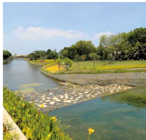
The Fengyuan Huludun Park Expo Site utilized its existing riverfront to create a “Floral Metropolis by the Water.”
