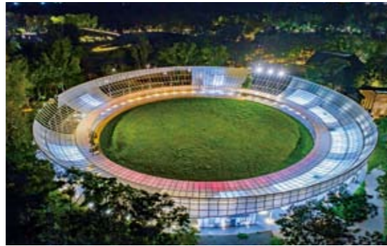
Houli Forest Expo Site tourist center removed the wall and exposed structural system to integrate it with the adjacent forest.
