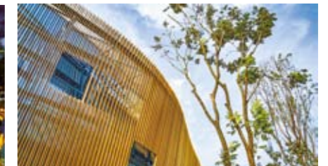
Blossom Pavilion A is an arch-shaped space surrounded by a metal grille, where visitors view changes in light and shade from different angles.
