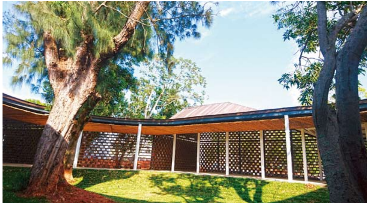
The Discovery Pavilion of Houli Forest Expo site coexists with the old tree on the site
