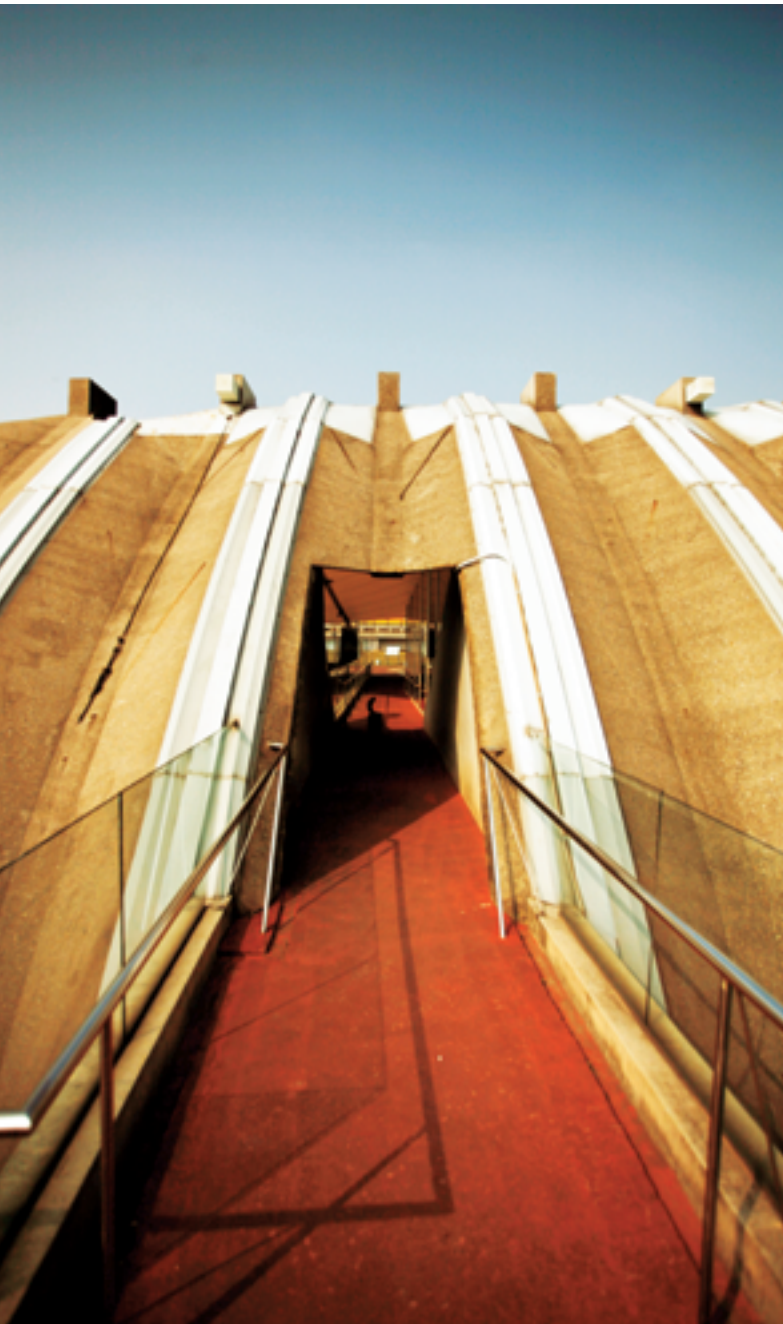
Building materials are used to redefine a traditional structure by applying a new skin and architectural design.
