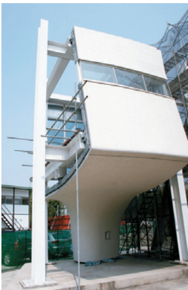
A pilot model on a 1/1 scale for construction execution.
