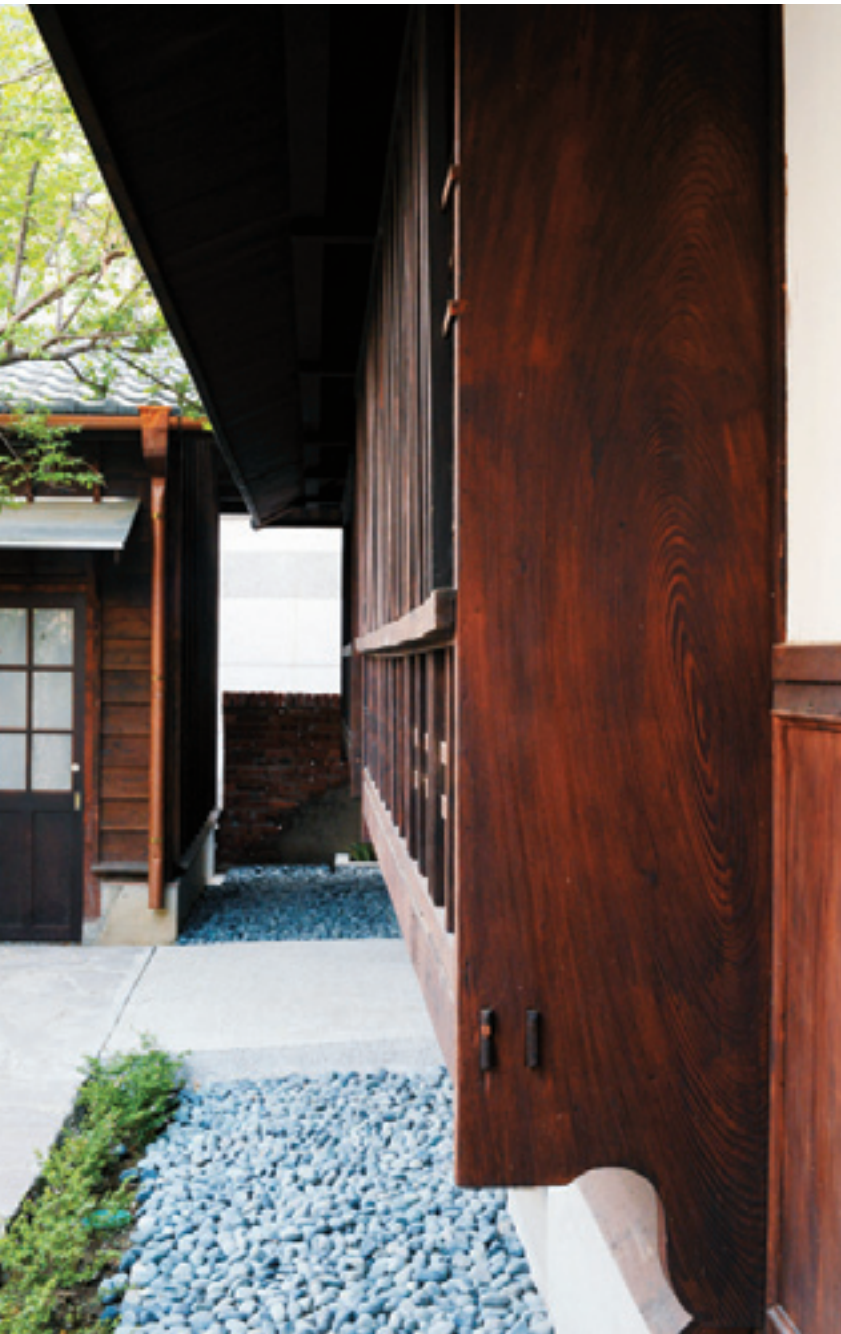
Police dormitory windows.
