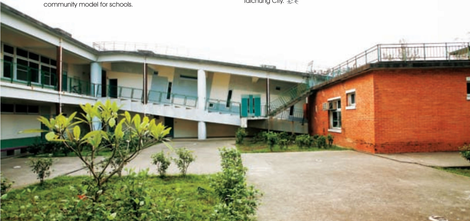
Students can experience different dimensions and structures within courtyard areas.
